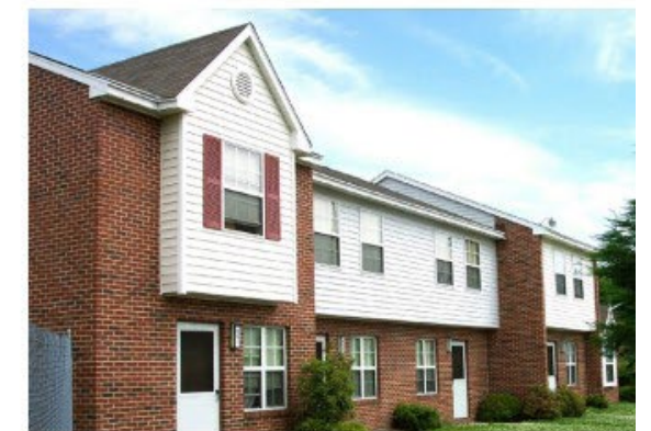
The newly renovated Lassiter Court Apartments in Newport News preserves much needed affordable housing in the area.
